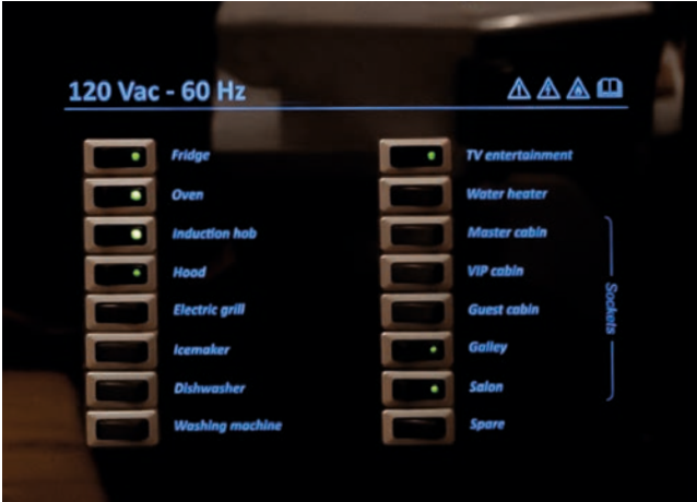
Circuit breakers for 120V consumers
